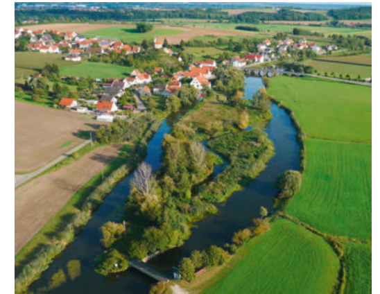
Wörnitz with millstream: Typical for the use of water power is splitting off into a millstream (waterway on left) and lower course. Water level is regulated by a low-head dam (in foreground).
