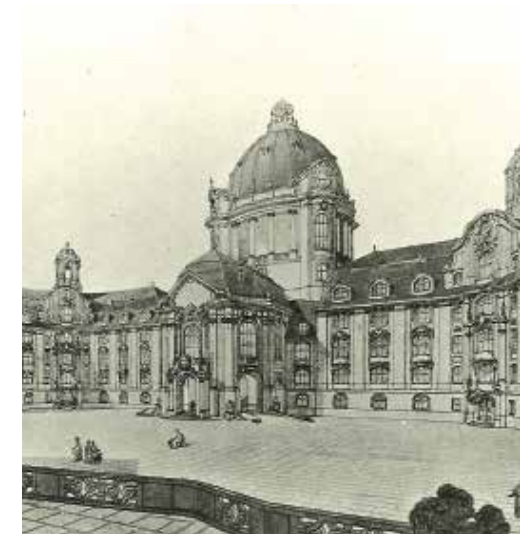
Suevite was used for the construction of the former Bavarian Ministry of Transport building in Munich.
