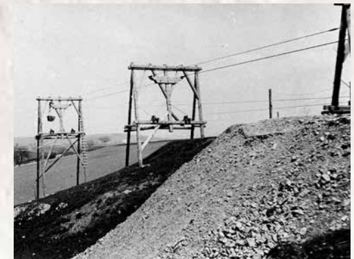
After 1924 the transport to Möttingen was done by cable rail
